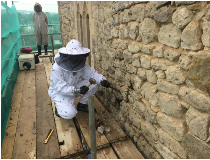
John the stonemason, making a start, by removing the first rag stone.
