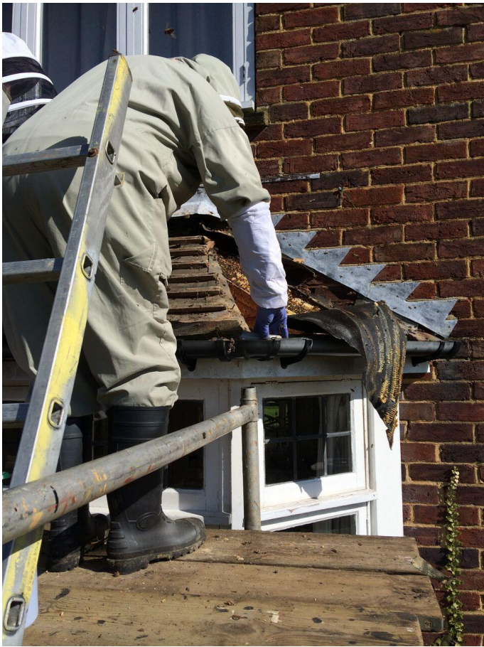
John removing the corner under felt.
